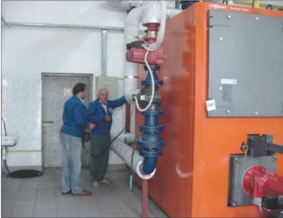
Employees at GIG's Laboratory of Work Environment Studies and Air Protection measure total pollutant emissions from a new gas boiler at the Barbara Experimental Mine at Mikołów, Upper Silesia.
